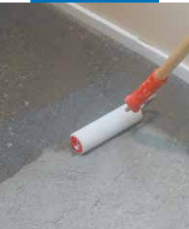
Applying Primer G with a roller
