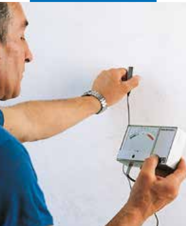
Checking plaster humidity
