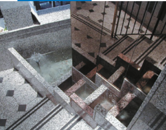
An example of an installation of a granite floor and wall with Keraquick + Latex Plus - Caesars palace in Merseyside - Liverpool (GB)
