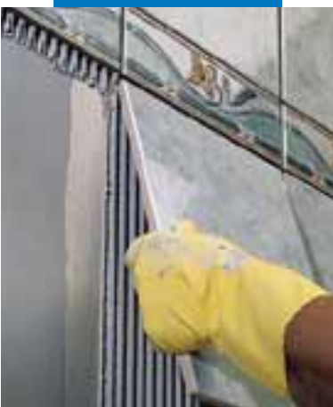
Installation of single-fired tile on wall render
