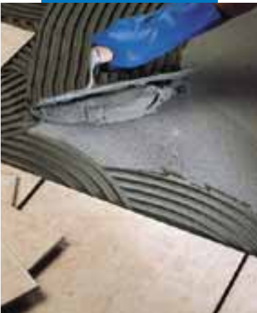
Installation of single-fired tile on floor
