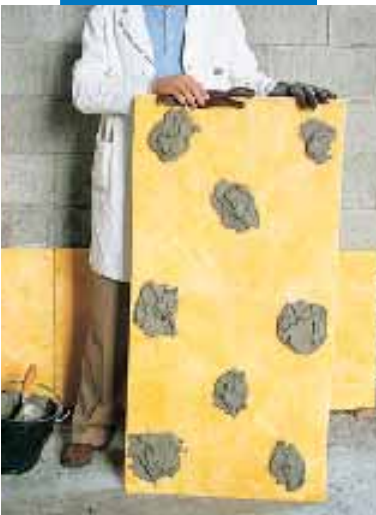
Spot-bonding insulating panels on untreated wall
